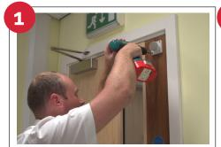
The Agrippa door holder is battery powered and wirefree. The device is installed at the top of the door.
