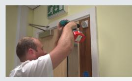
Align the keeper plate with the magnet face.
