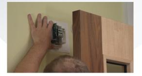
Use the paper template supplied to drill holes in the wall.
